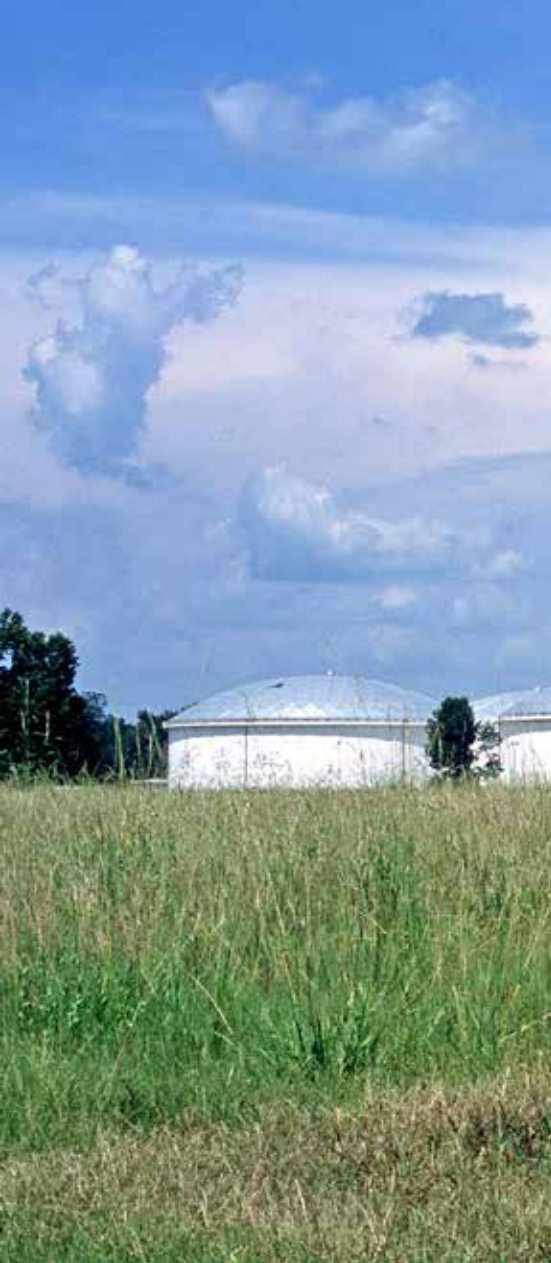
Photo courtesy of Colonial Pipeline Company
