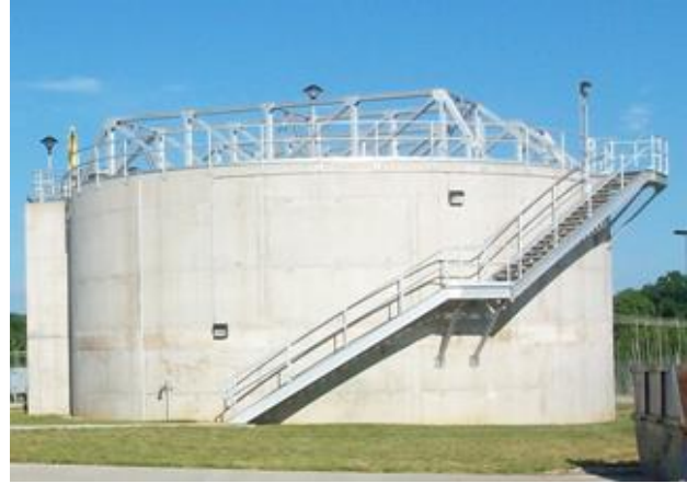
Figure 8-2 Example Gravity Thickener Installation
