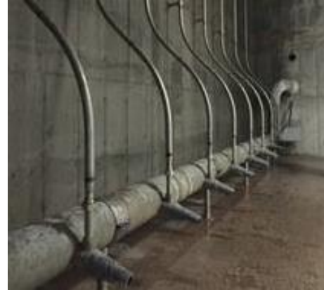
Figure 8-14 Autothermal Thermophilic Aerobic Digestion Aeration System
