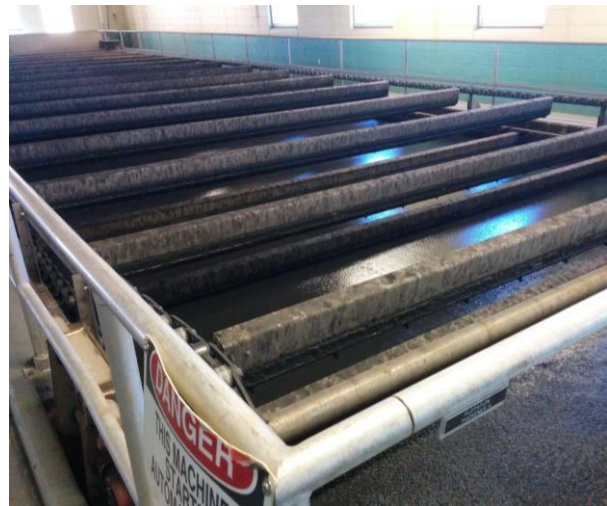
Figure 8-5 Example DAF Thickening Installation
