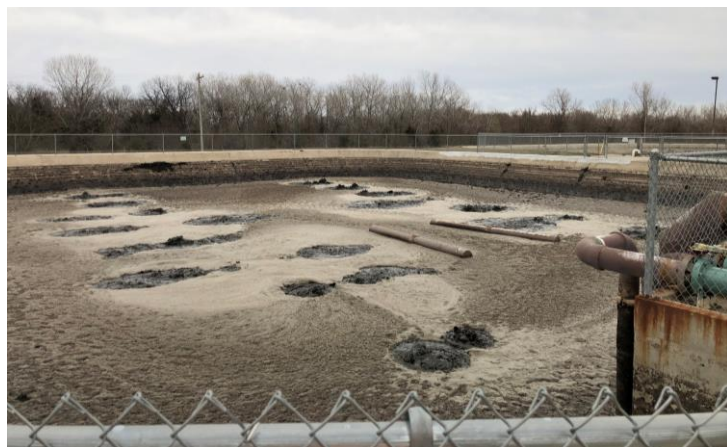
Figure 8-12 Aerobic Digester
