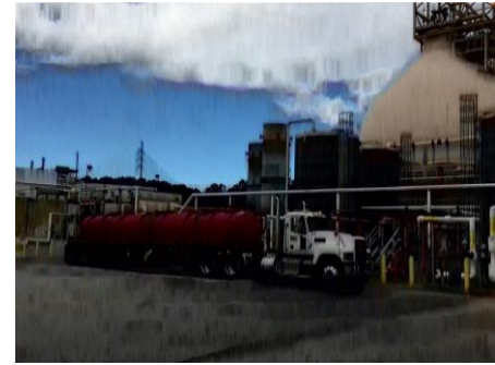
Figure 10-5 FOG and HSW Receiving at F. Wayne Hill WRC in Gwinnett County
