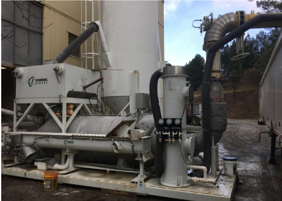
Figure 8-21 Example Lime Stabilization Installation in Atlanta, Georgia
