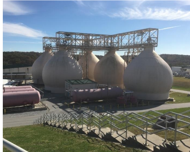
Figure 8-15 Anaerobic Digesters in Gwinnett County
