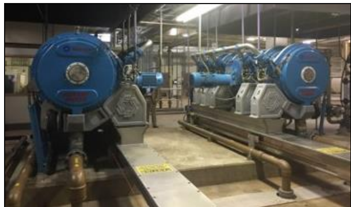
Figure 8-9 Example Rotary Press Installation
