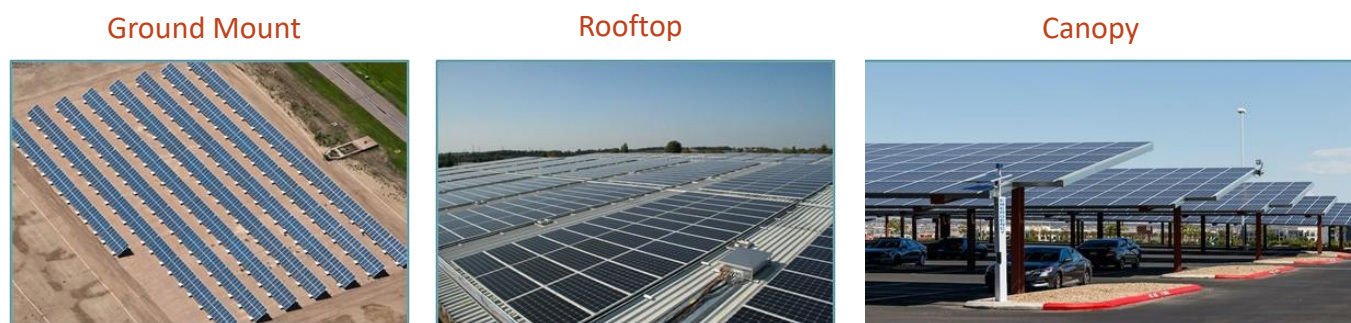
FIGURE 10 – IMAGES OF SOLAR MOUNTING CONFIGURATIONS
